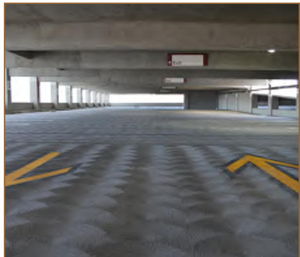
Rotary Swirl Finish for Parking Decks
