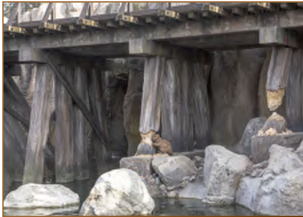
Concrete Simulating Aged Wooden Trestle Bridge
