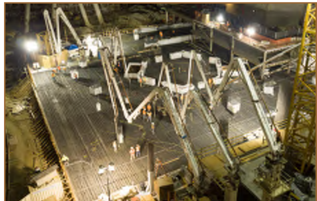
Placing Booms on a 9,600CY Mat Foundation Pour at the New Century Plaza, Century City, CA
