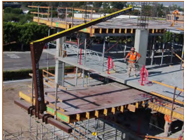
Formwork Table Caddy
